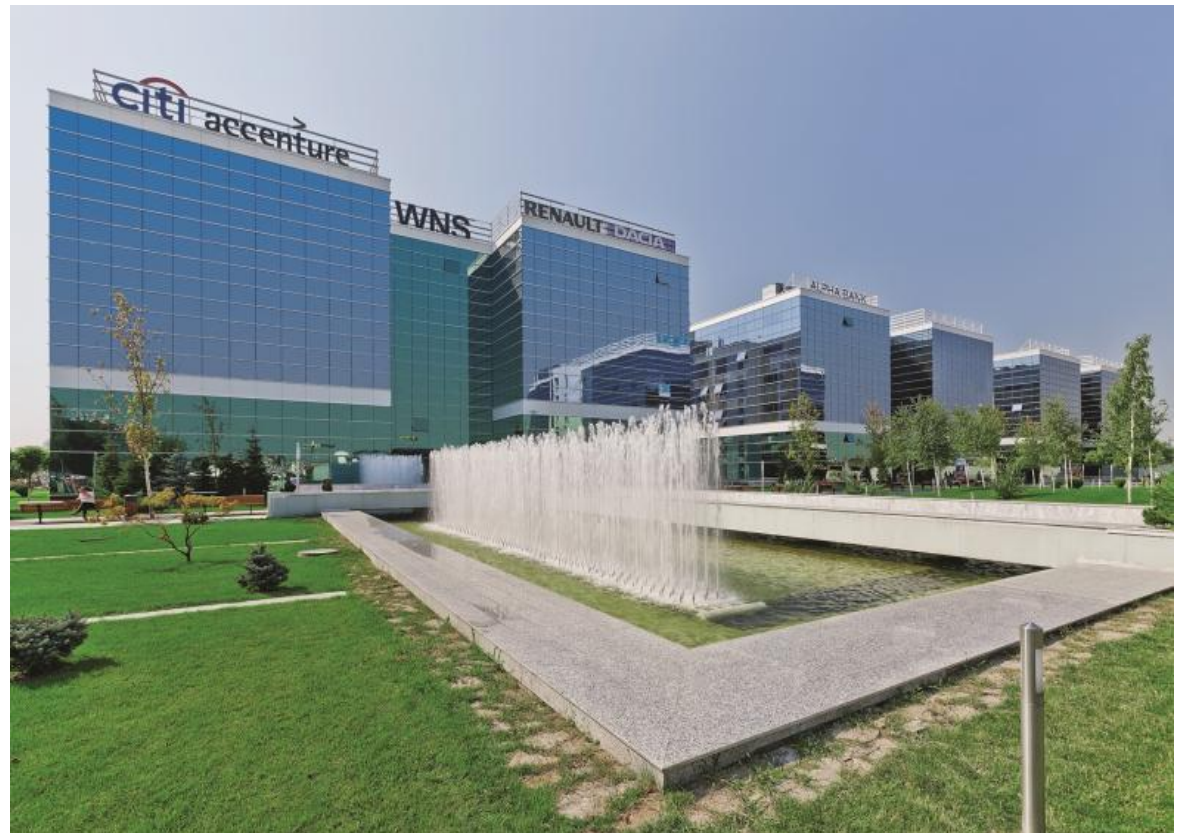
West Gate Business Park
